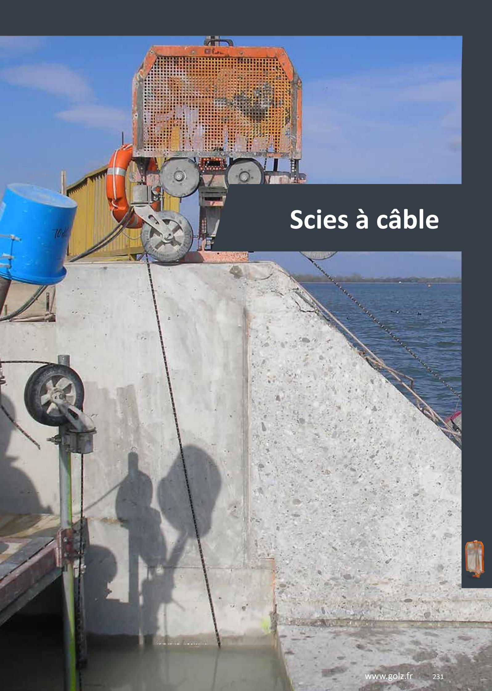
A large orange cable saw machine is mounted on a boat, positioned to cut through a concrete pier. The machine has a protective metal cage and several pulleys. A thick steel cable runs from the machine down the side of the pier. In the background, there is a body of water and a clear blue sky. A blue bucket is visible on the left side of the boat. The machine is cutting through the concrete, and a shadow of the operator is cast on the pier's surface.
